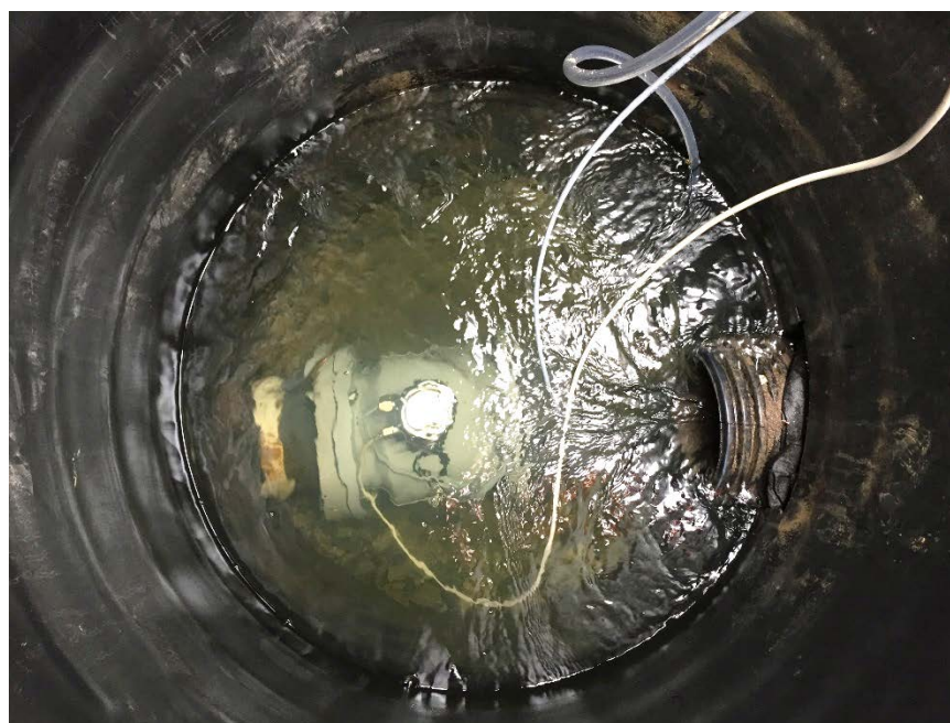
Figure 4. 8-inch diameter Waterflux 3000 flowmeter in JBT11 manhole
