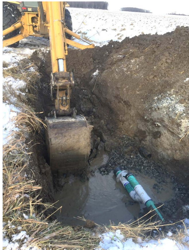
Figure 1. Installation of a pipe trap and manhole at JBT02
