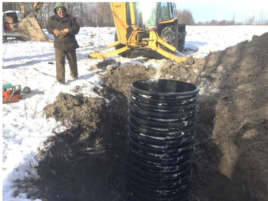
Figure 2. Lowering manhole into place over tile drain piping
