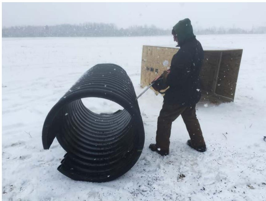
Figure 3. Cutting notches in manhole for incoming and outgoing pipes
