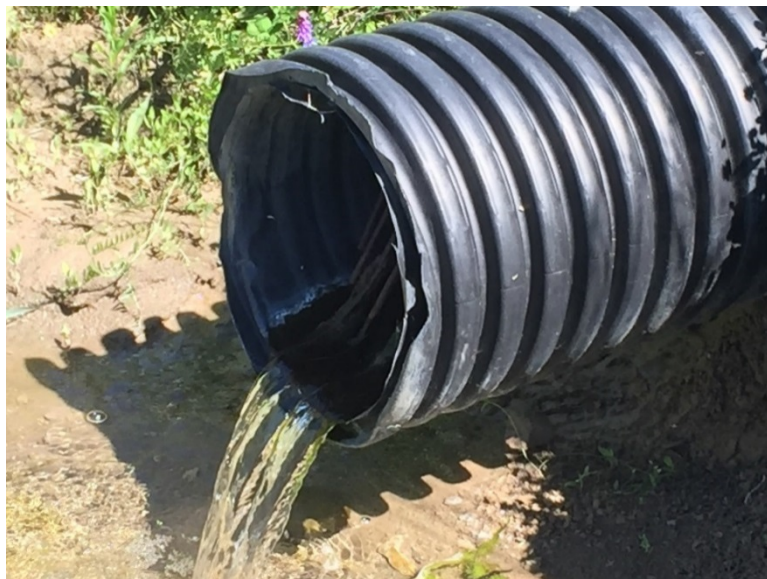
Figure 7. JBT06 outfall (12-inch diameter)
